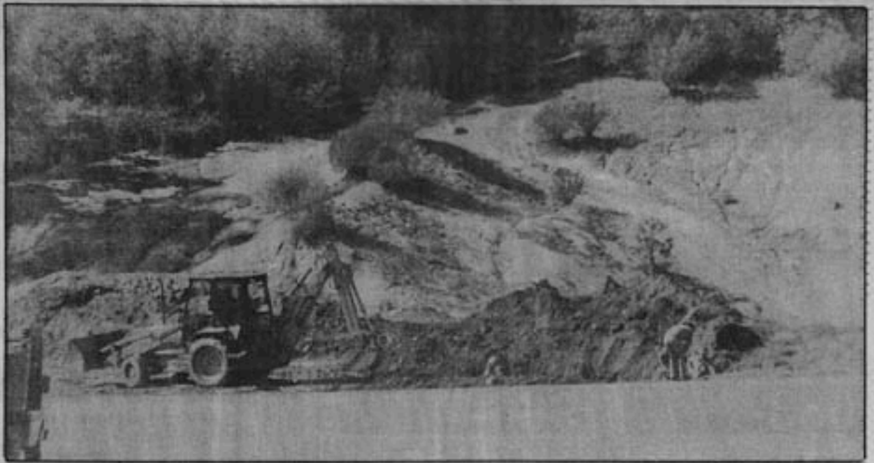
PRELIMINARY WORK ON INTERSECTION: Madera County Road Department is working on drainage at the "Crazy Y" intersection in North Fork. According to a
